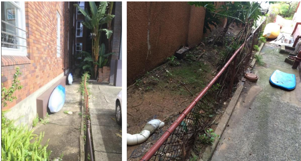
Figure 15: Previous fence located between 4 and 6 Billyard Avenue. Photographs were provided by the applicant and dated to September 2014.
