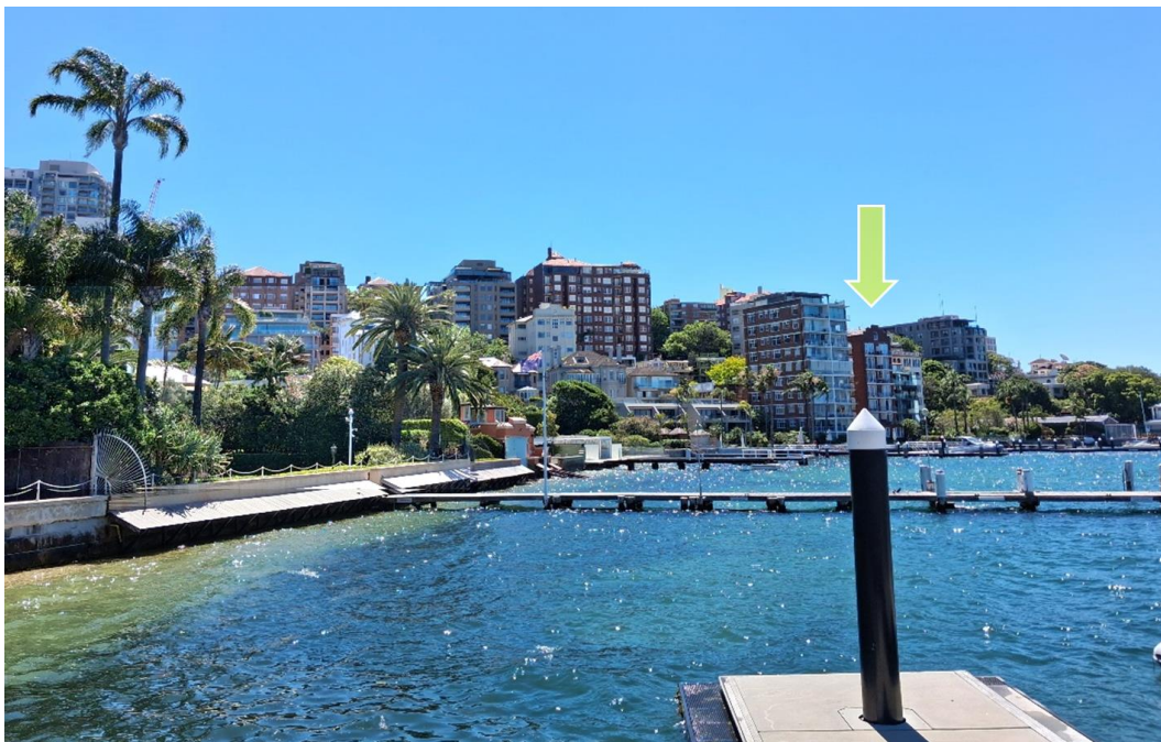
Figure 10: Subject site (as indicated) viewed from the Elizabeth Bay Marina located to the south
