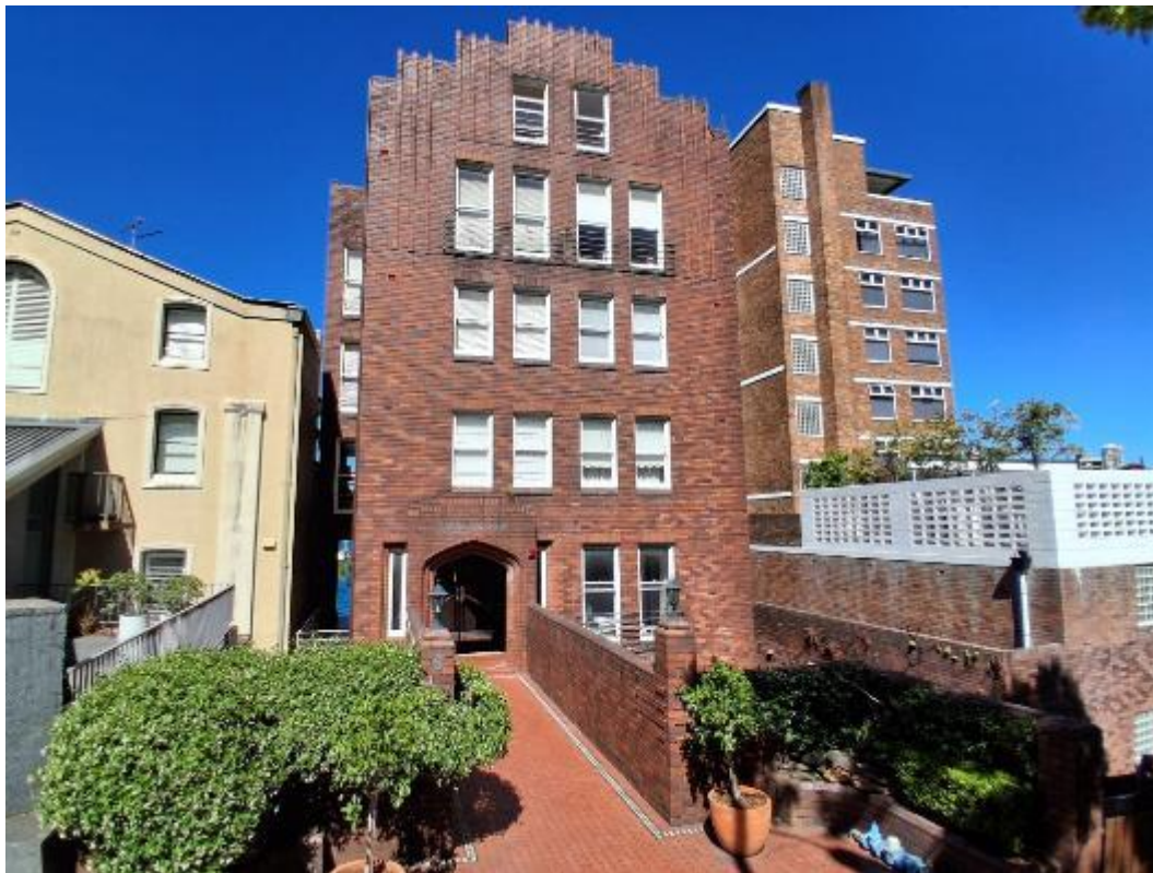
Figure 3: Site viewed from Billyard Avenue
